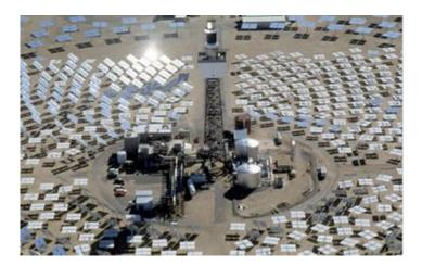
Using electricity generated at Ivanpah means displacing more than 400,000 tons of carbon dioxide (CO2) each year and decreasing water use by 95 percent when compared with wet-cooled solar plants.
